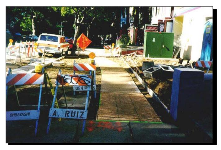
Temporary ramps and boardwalks ensure smooth continuous surface
