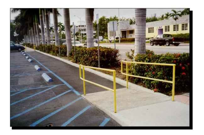
Handrails Should Not Protrude into the Pedestrian Route (Must comply with ADAAG)
