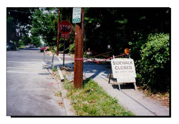
This barrier does not provide adequate warning and rerouting signs
