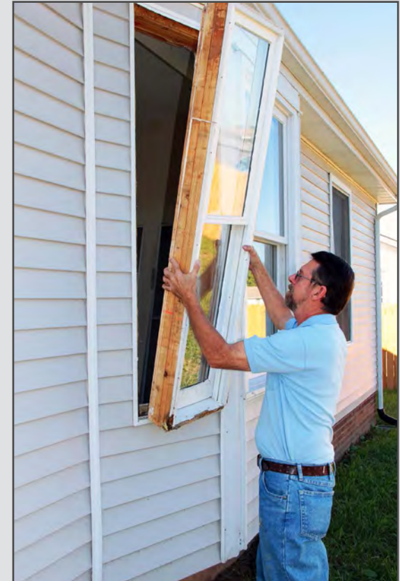
NYC found a creative way to finance energy retrofits.
