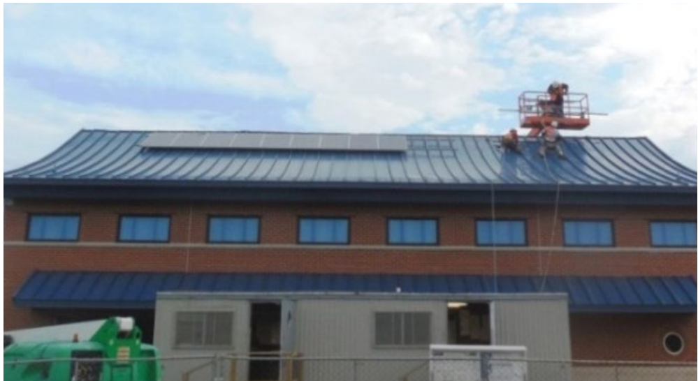
Installation of solar panels at Metro's net zero energy stormwater facility.
