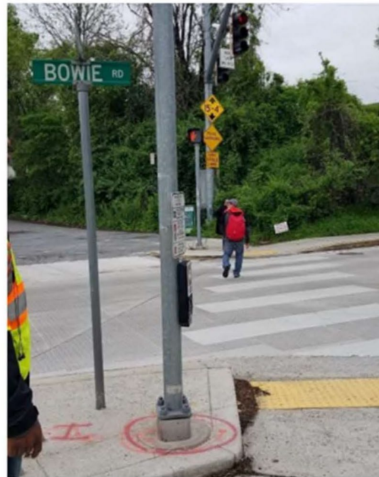
Insufficient crosswalk marking contrast
