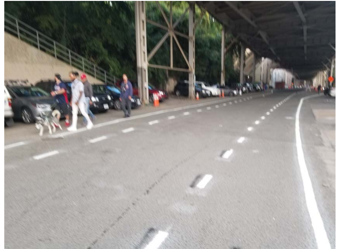
Water Street NW
