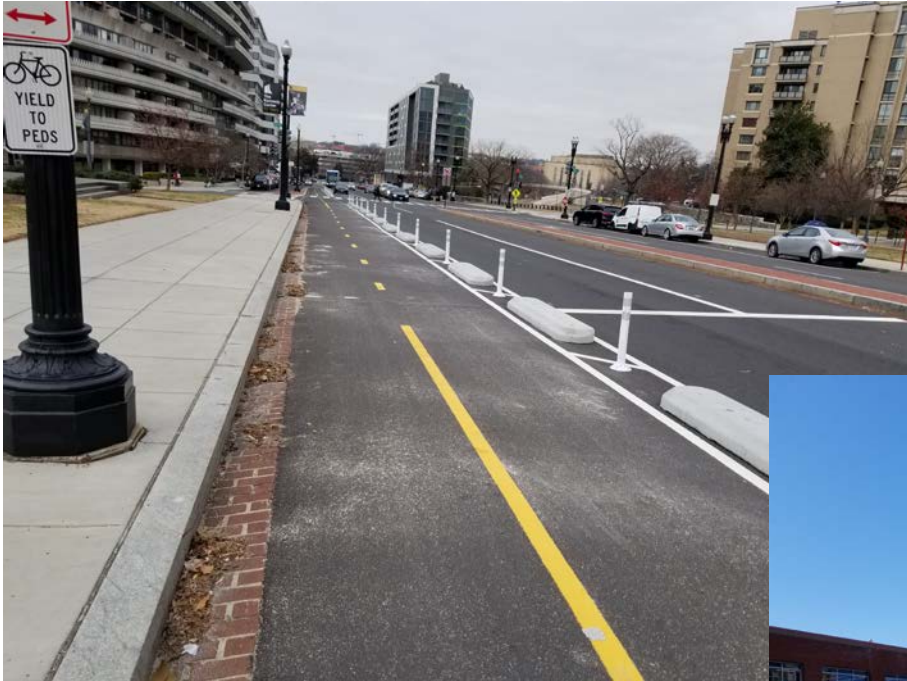
Virginia Ave NW
