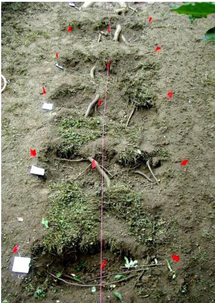
Six excavated "windows" into the ground
