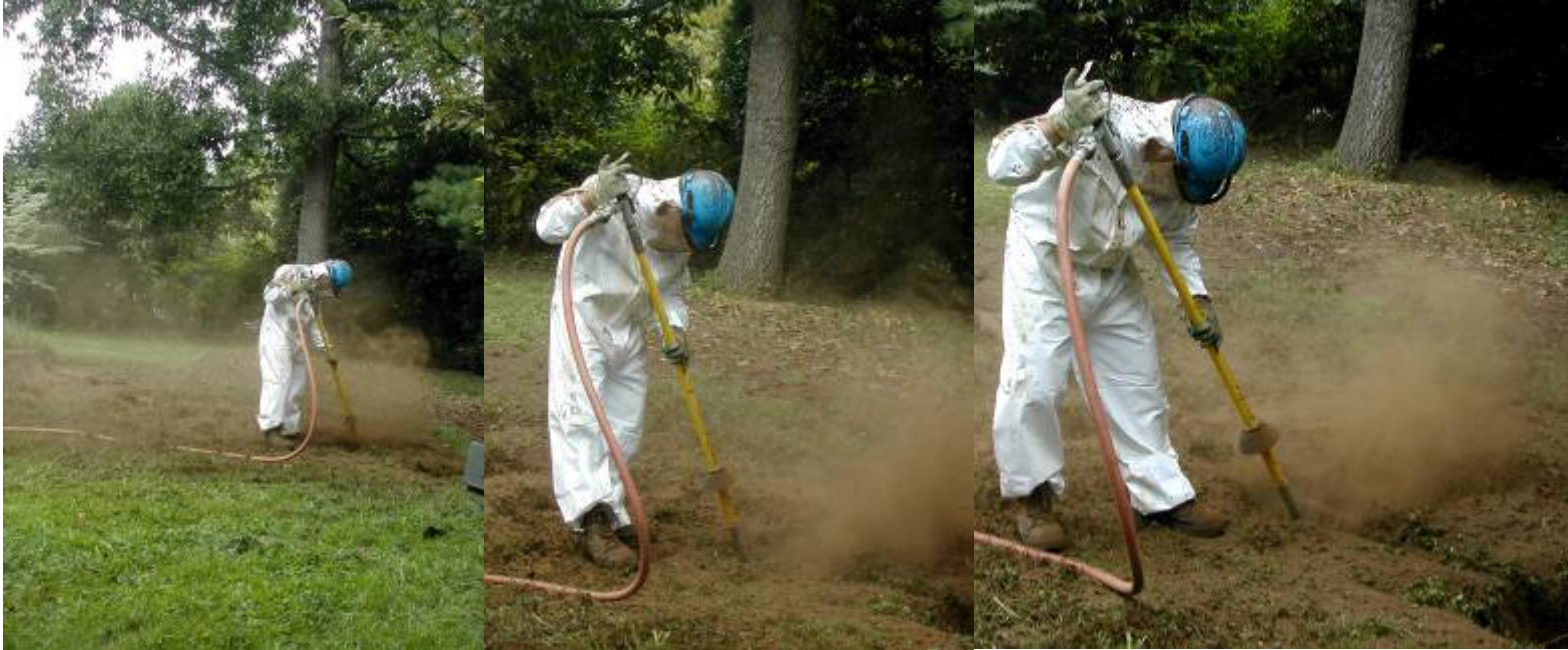
Excavating the Soil using the Air-Spade high-velocity Air Gun
