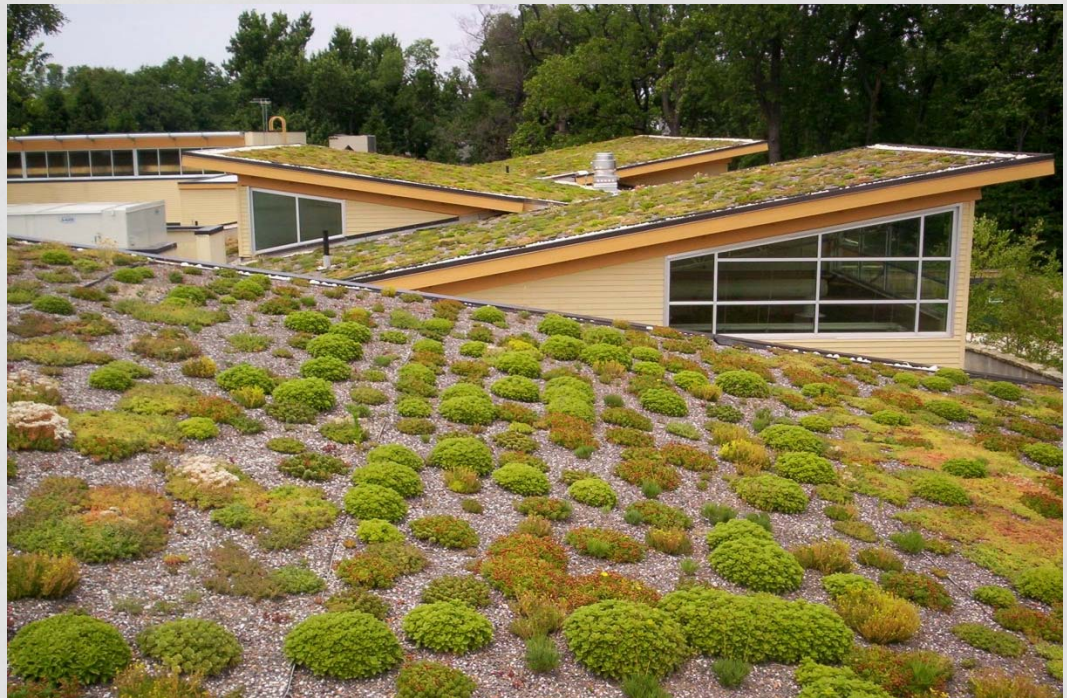
Green Roof at Walter Reed Community Center Photo Credit: Arlington County
