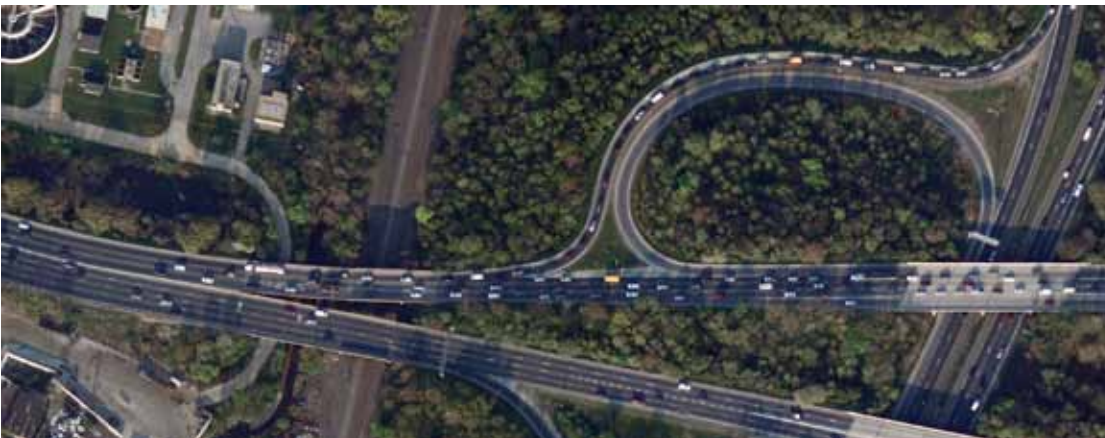
Photo Set Two: These photographs show the 2005 (top) and 2011 (bottom) configuration of the DC 295 bridge across the Northeast Corridor railroad right-of-way; note the absence of a significant merge lane in the 2005 photograph, and the friction that caused for southbound traffic on DC 295.
