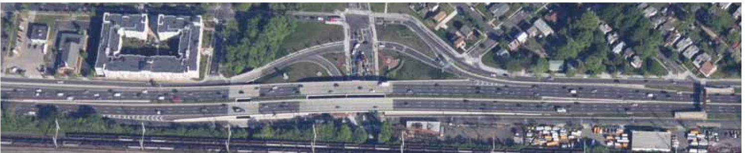
Photo Set One: This pair of photographs show the reconfiguration of the Nannie Helen Burroughs Ave NE interchange between 2005 and 2011. Note the lengthened deceleration lane to the right side of the 2011 image.
