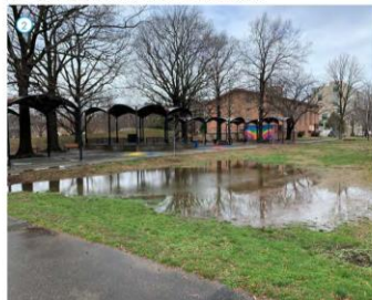
Existing topography results in flooding during storms
