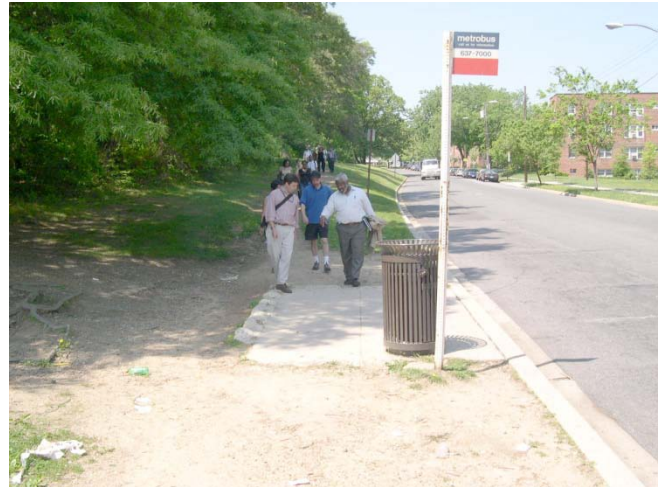
Figure 1: Missing sidewalk near Ft. Totten Metro
