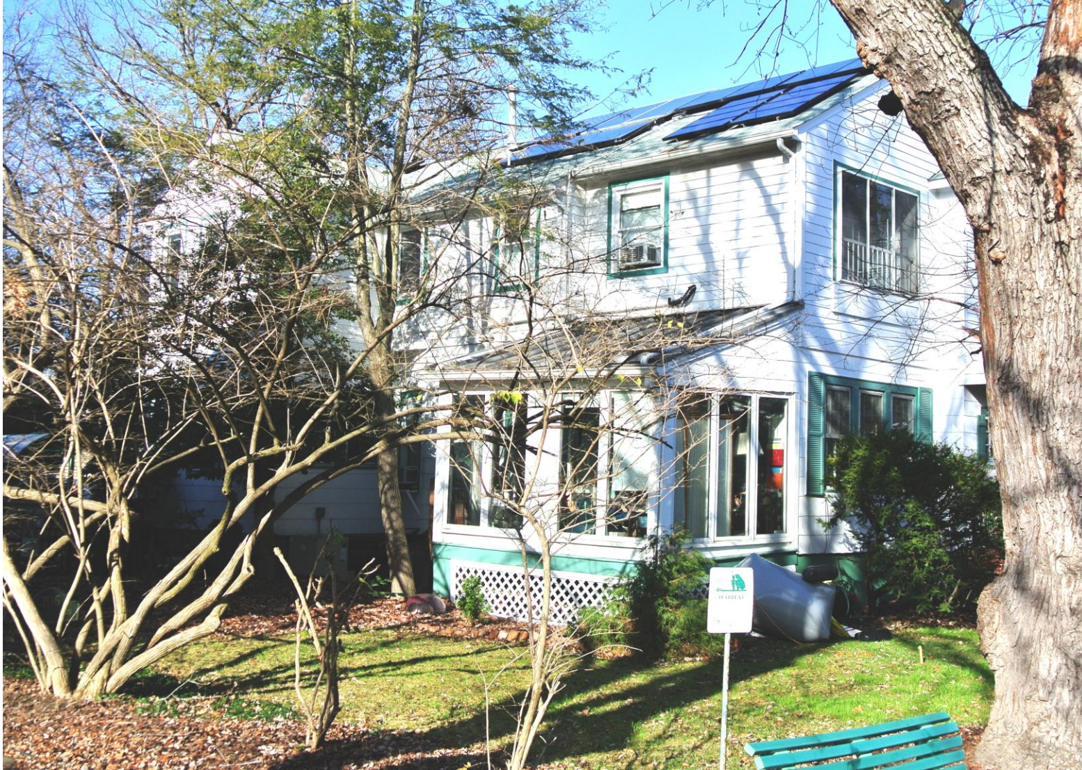
SKLAR ARLINGTON 1921 SEARS KIT HOME: R-38 insulation, low-e double-paned windows, thermal barrier paint under the attic roof, LEDs, Energy Star appliances, solar water heating, geothermal heating & cooling, PV with battery bank, electrochromic glass, LEDs, etc.
