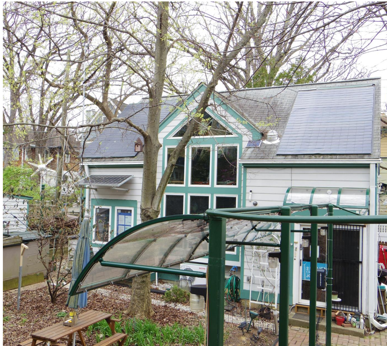
StellaGp office building: R-50 insulation, super-insulating windows, solar daylighting, PV Driven ceiling fans, PV shingles, small wind turbine, hydrogen fuel cell all tied to a web-enabled battery bank
