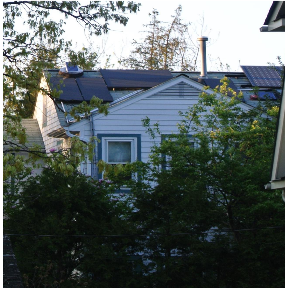
SKLAR HOUSE – SOUTH FACE (WEST SIDE OF ROOF)
