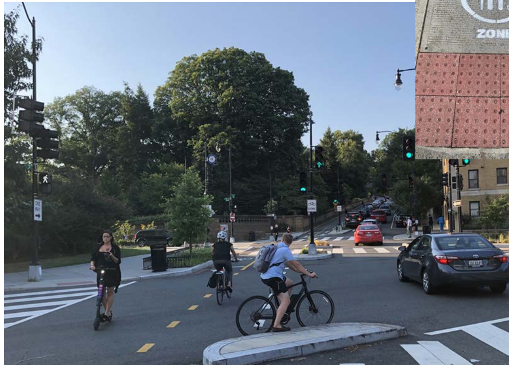
14 th Street NW Protected Bike Lane
