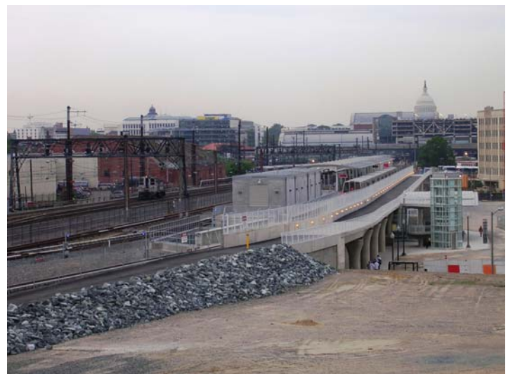
The New York Avenue Metro Station Incorporates a Shared- Use Path and Bicycle Parking
