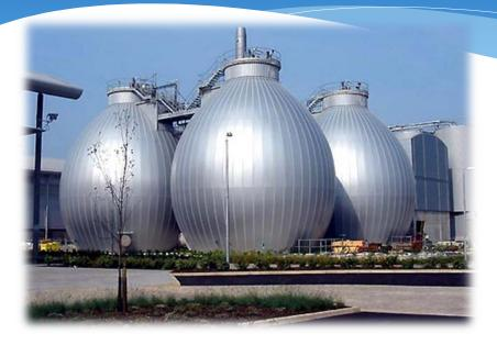
Co-combustion of dewatered sewage sludge from the County's WWTP (which is adjacent to the WTE Site) will eliminate the need to construct egg shaped anaerobic digesters.
