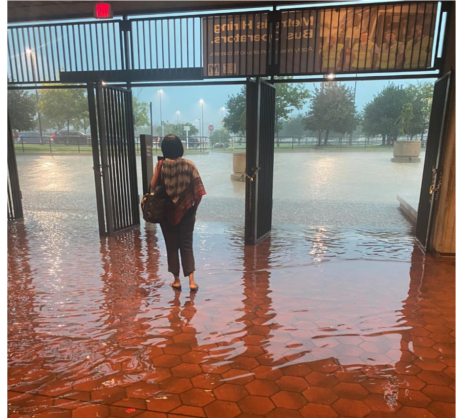
Flooding at Greenbelt Metro Station, August 2022. Source: Washingtonian
