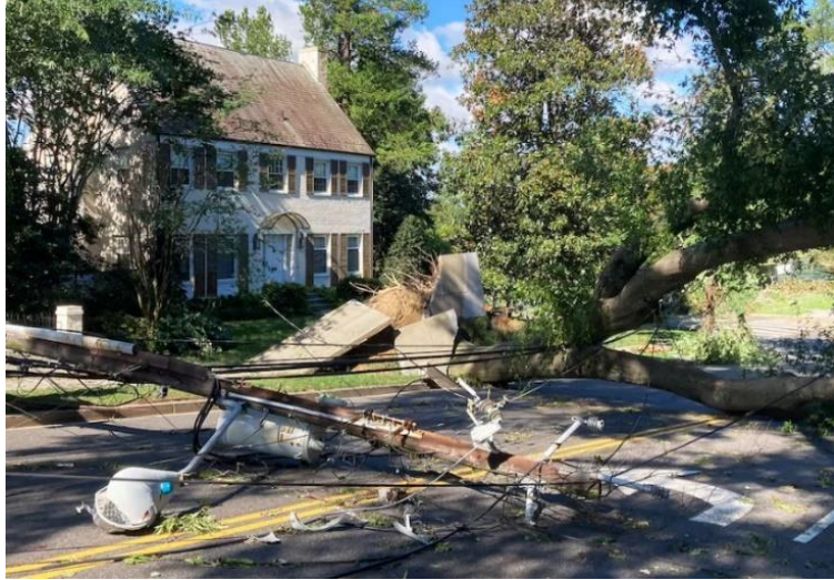
Fallen trees and broken power lines after the severe storm in 2023. Source: The Washington Post.
