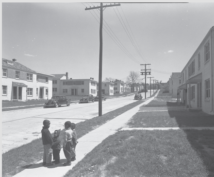
Barry Farms Housing Development, 1944.
