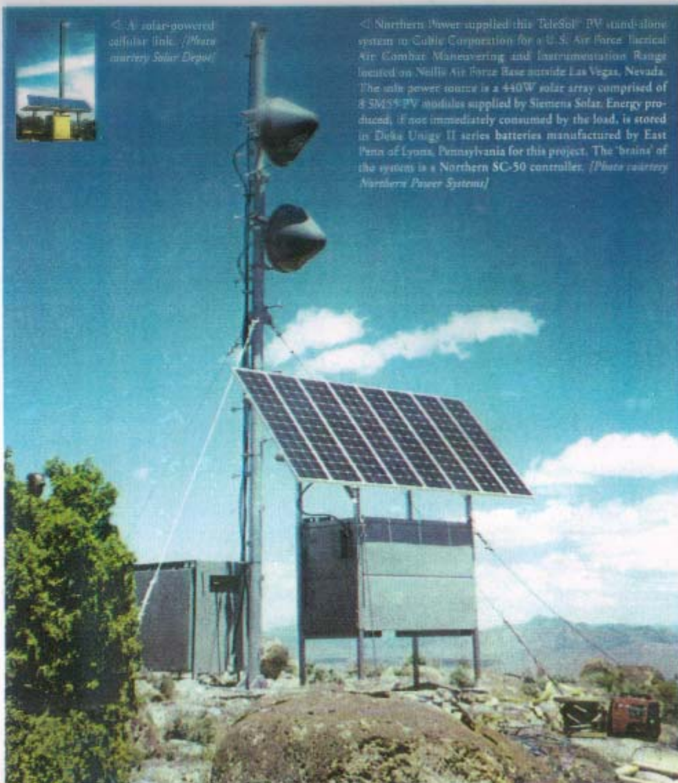
◀ A solar-powered remote telemetry system provided by Solar Depot, San Rafael, California. This is a common application for photovoltaics. [Photo courtesy Solar Depot]
