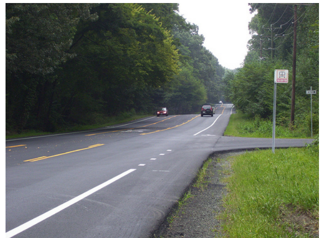
Figure 12: Lawyers Road After Road Diet
