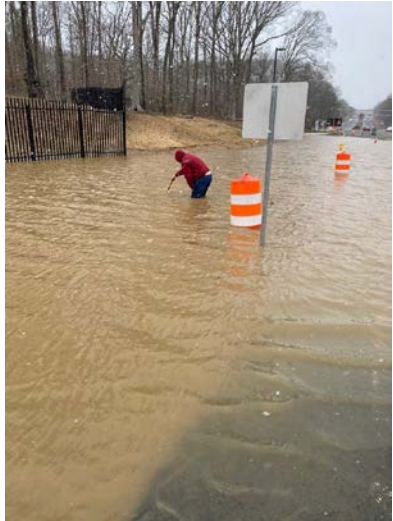
Main Gate Flooding at Quantico
