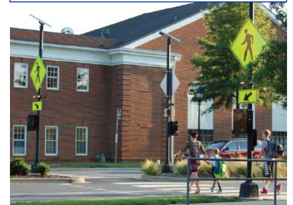
Rectangular Rapid Flashing Beacon
