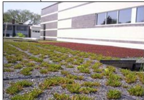
District of Columbia's Trinidad Recreation Center has a green roof that reduces heat island and is estimated to reduce 81,000 gallons of stormwater a year.
