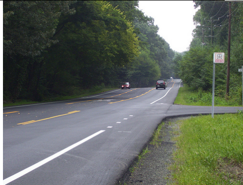
Figure 1044: Lawyers Road After Road Diet
