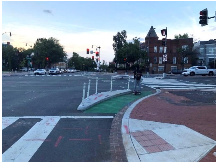
Figure 31: Partial Protected Intersection/TPB/Michael Farrell
