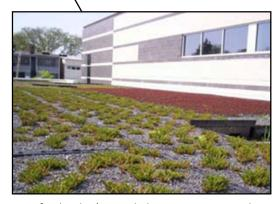
District of Columbia's Trinidad Recreation Center has a green roof that reduces heat island and is estimated to reduce 81,000 gallons of stormwater a year.
