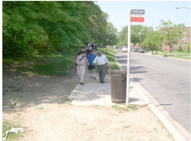
Figure 55: Missing Sidewalk/TPB/Michael Farrell
