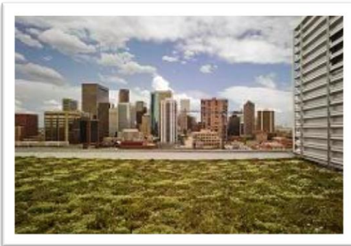
Figure 18: A 1,711 square foot green roof was installed on the area of roof that connects Potomac Yard One and Two in Arlington, Virginia.
