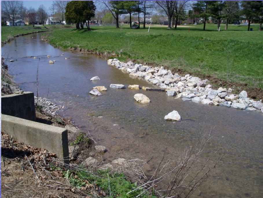
Rock deflector on Willis Run installed by inner-city high school students
