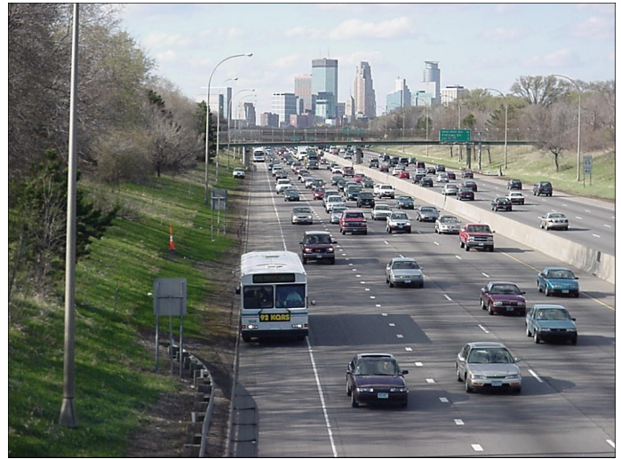
In the Minneapolis-St. Paul metropolitan area, buses are able to use the shoulder of major highways to bypass congested travel lanes.
