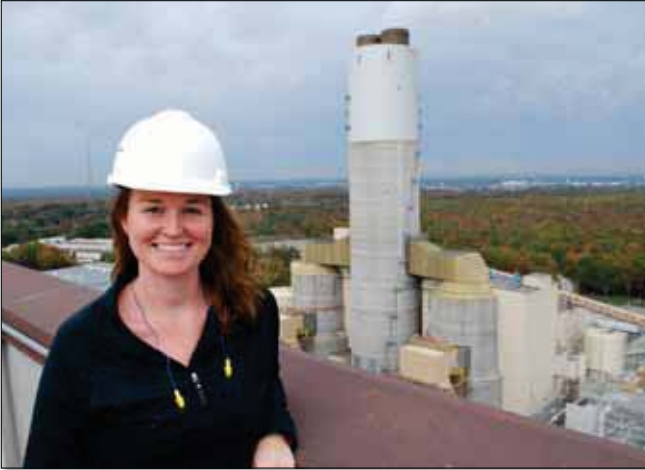
In response to a 2006 Maryland air pollution control law, Constellation Energy built this scrubber at its Brandon Shores coal-fired power plant and hired 32 workers in part to run and monitor the scrubber. Among those hired was chemical technician Melissa Sampson (above).
