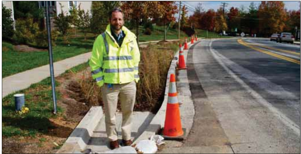
Steve Shofar, Chief of the Watershed Management Division for Montgomery County, Maryland, stands inside a "bump out"—a grassy area built along the side of the road to filter rainwater—of which Montgomery County plans to build hundreds of to meet the Chesapeake Bay pollution limits.
