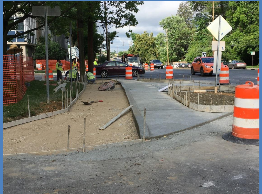
Construction of Spring Street Separated Bike Lanes
