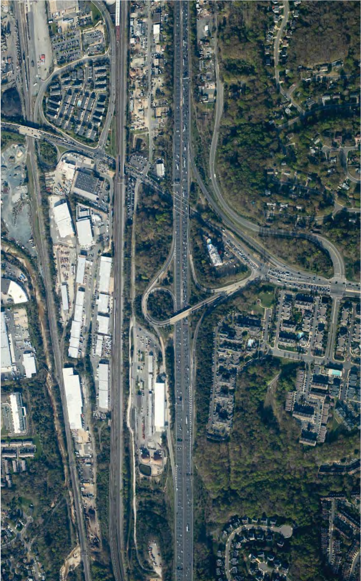
Photographs: The 2014 photo above shows eastbound congestion on the outer loop of the Beltway at the Van Dorn St Interchange. During the 1999 survey (pre-construction), free-flow conditions were typically found here.
