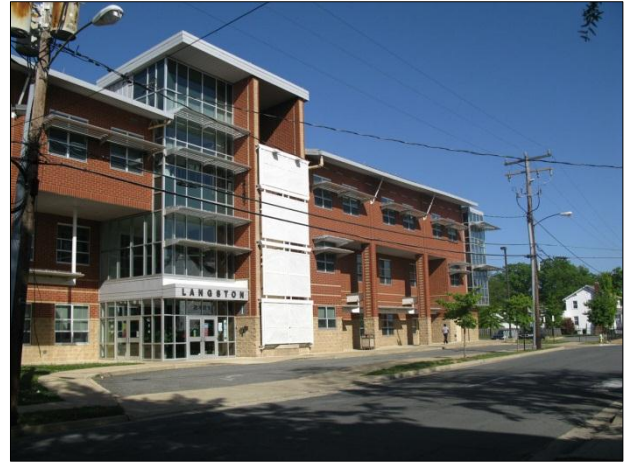
Figure 23: The Langston High School and Langston-Brown Community Center's passive survivability features include shades over windows and two 11,000-gallon cisterns, one of which is behind the white screen.
