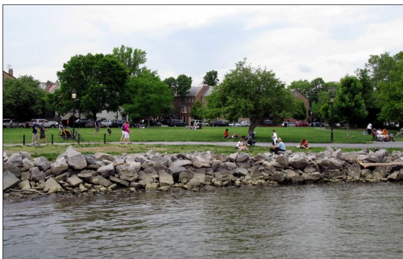
Figure 12: This waterfront park in Alexandria, Virginia, along the tidal part of the Potomac River, is vulnerable to flooding.
