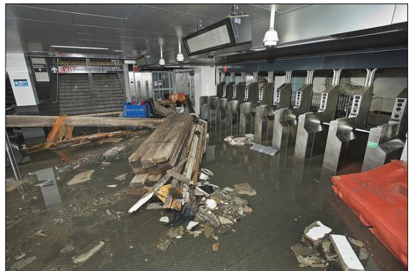
Figure 16: Superstorm Sandy in October 2012 showed how powerful storms can damage both aboveground and underground transit facilities.
