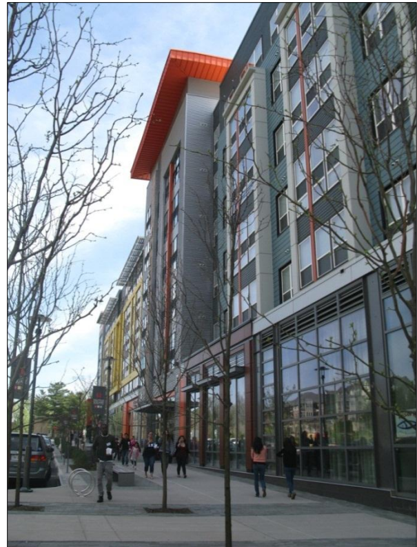
Figure 20: Halstead Square, about one block from the Dunn Loring Metro station, offers more than 1,000 apartments and lofts and over 100,000 square feet of commercial space.
