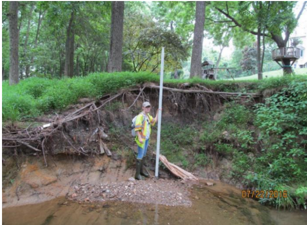
Brittenford, Before Restoration
