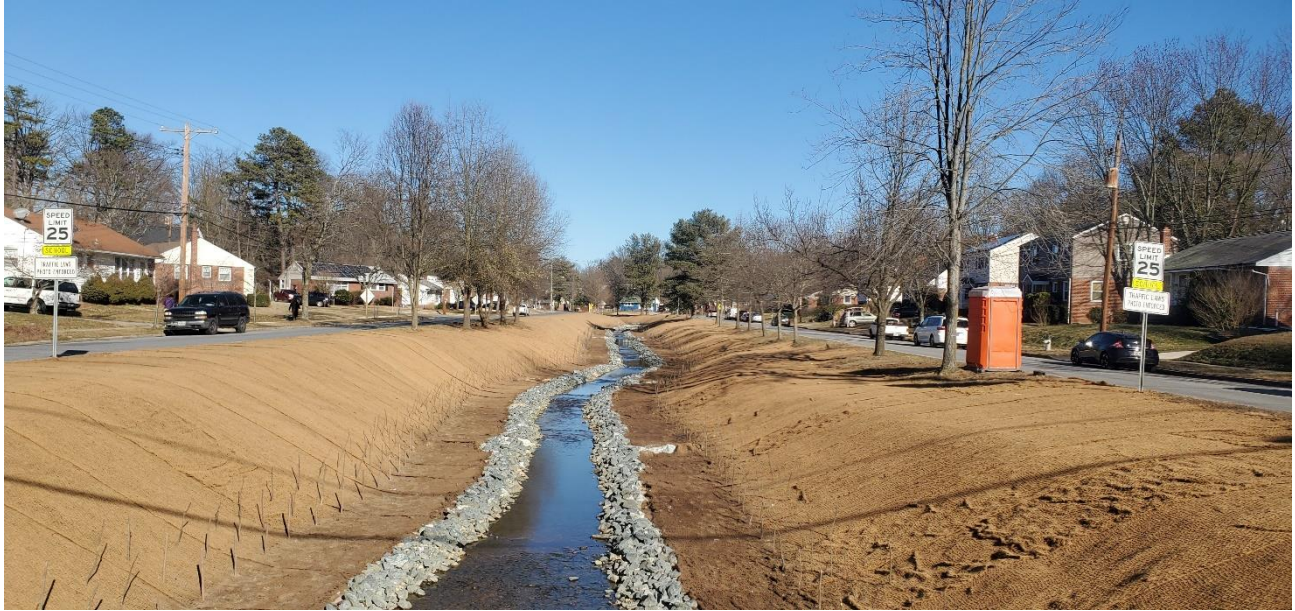
Briers Mill Run, After Restoration
