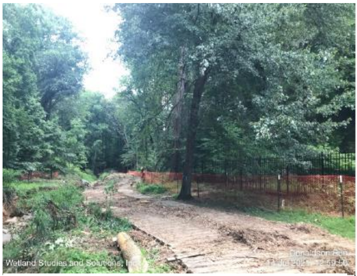
Example of saving trees during construction of the Donaldson Run Tributary B Stream Restoration Project in Arlington County. Access to the site was adjusted to save a tree important to the landowner. (Wetland Studies and Solutions, Inc.)
