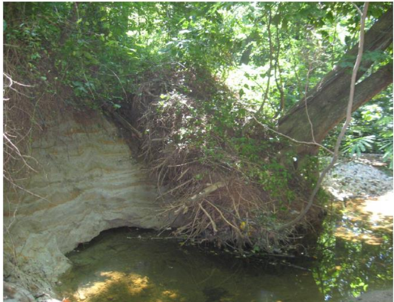
Before restoration, streambank erosion in this section of Powell's Creek in Prince William County led to loss of mature trees. (Prince William Department of Public Works)
