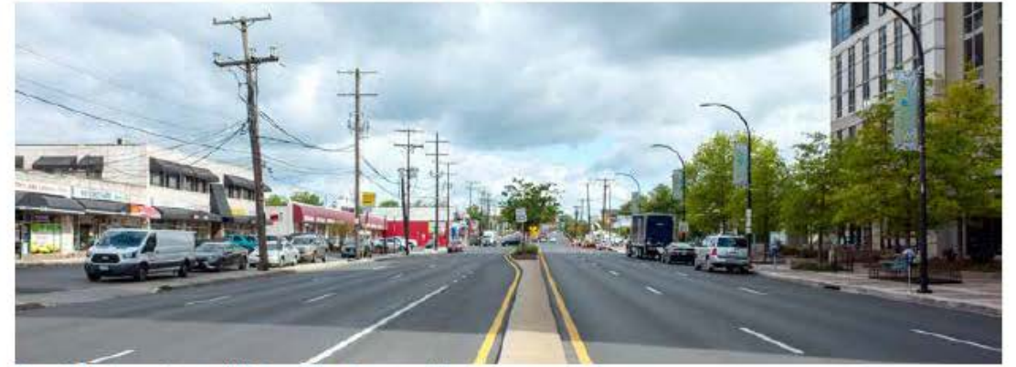
Figure 2-14. Georgia Avenue (MD Route 97) in Downtown Wheaton
