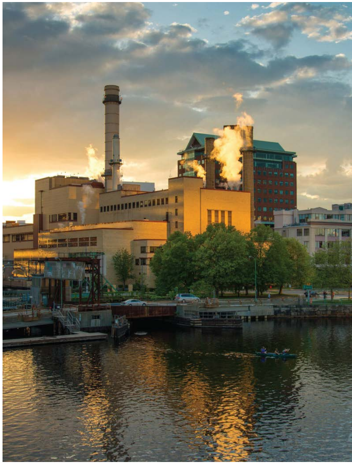
Kendall Cogeneration Station – District Energy Boston, Cambridge
