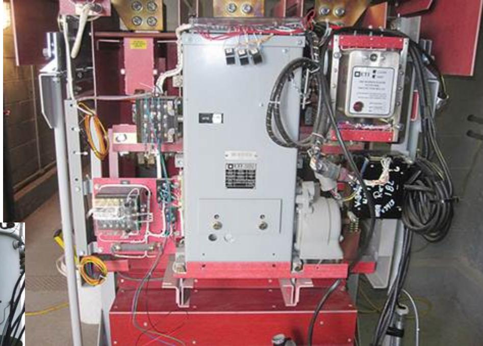
Retrofitted conEdison network protectors (2-Way Communication Relays)
