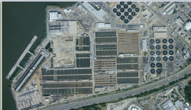
Blue Plains Advanced Wastewater Treatment Plant
