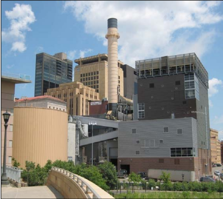
Figure 9. Biomass CHP Plant in Downtown St. Paul, Minnesota
