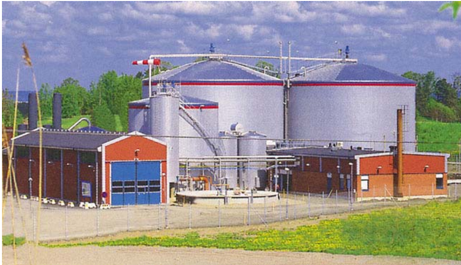
Figure 10. Biogas Production Facility in Linköping, Sweden
