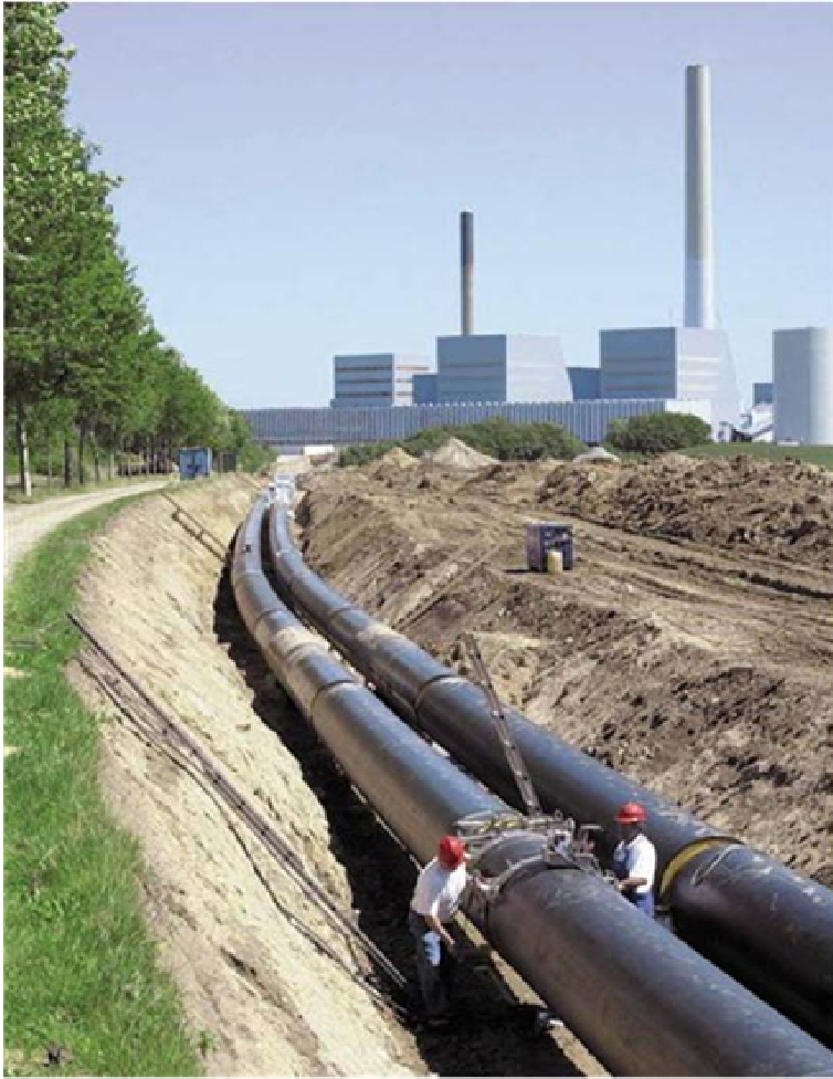
Figure 6. Long Distance Heat Transmission
