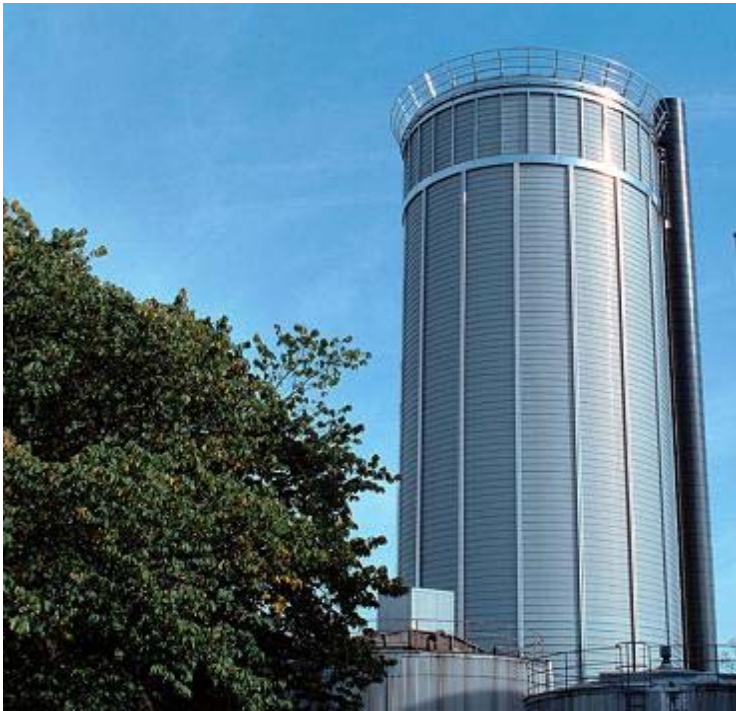
Figure 15. Hot Water Accumulator
