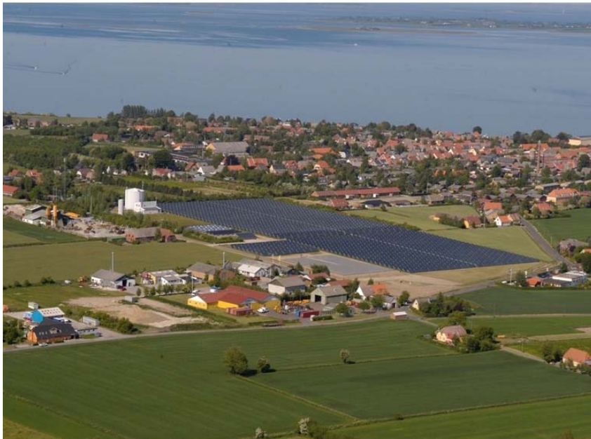
Figure 11. Solar Thermal Array for District Heating in Marstal, Denmark
