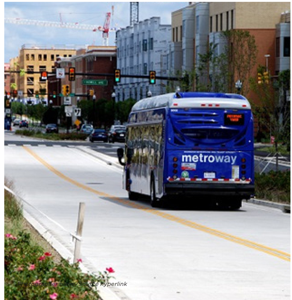
FIGURE 5 MEDIAN RUNNING PORTION OF THE CRYSTAL CITY POTOMAC YARD TRANSITWAY
