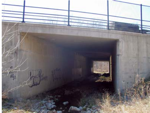
Photo A2.1. Wildlife Crossing in Fairfax County, Virginia.
