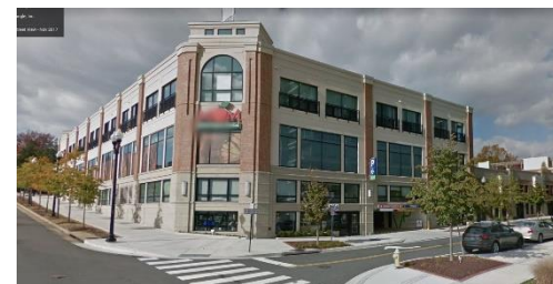
Liner Apartments Low-rise (Spout Run)
