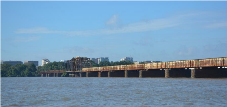
Long Bridge between D.C. and Virginia. (DDOT, 2020)
