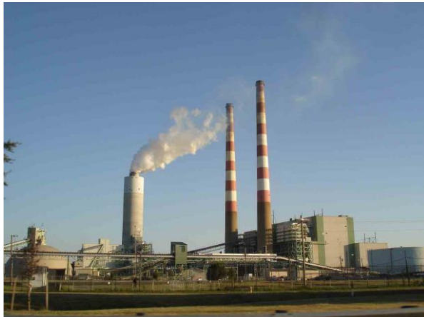
Wet Scrubber Installed at the Morgantown Coal Plant - 2009
