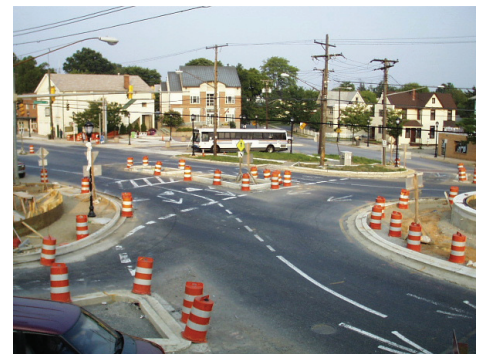
Mount Rainier, Prince George's County MD, roundabout on Route 1, a Maryland state highway. Roundabouts are considered the most effective technique for lowering vehicle speeds and reducing pedestrian crashes. Source: Retting et al., 2003.
