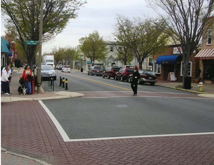
Alexandria uses curb extensions to reduce crossing distances for pedestrians on Mt. Vernon Avenue.
