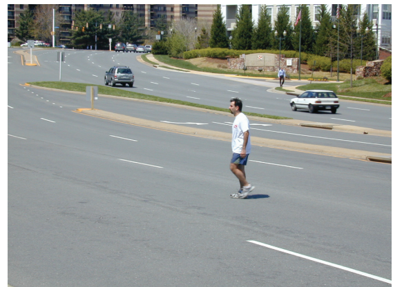
Wide roads and long distances between intersections in Tysons Corner, Fairfax County.
