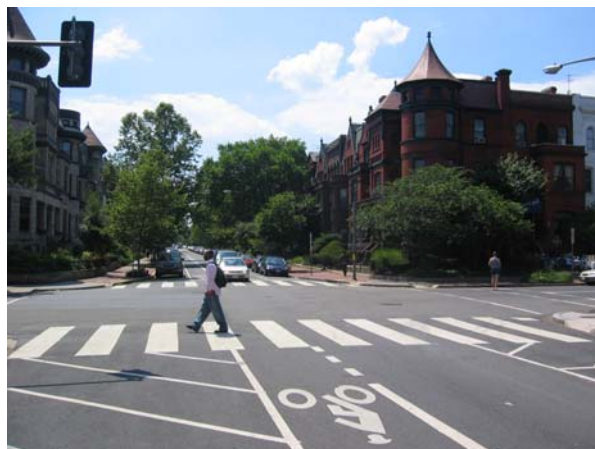
The Urban Core has well-developed facilities for Walking and Bicycling
