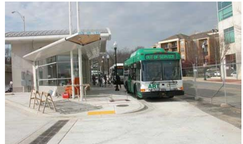
The Shirlington Transit Station, currently under construction in Arlington, VA.
