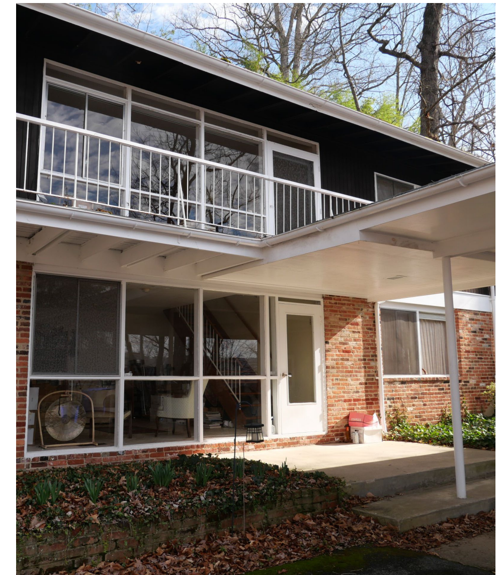
7205 MacArthur Boulevard, part of Potomac Overlook Historic District
