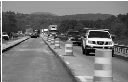
I-81 Pavement Project
