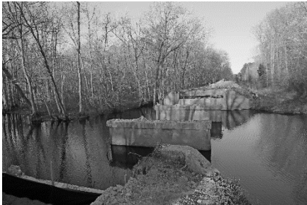
Carson Road (Rte 703) Bridge Replacement
