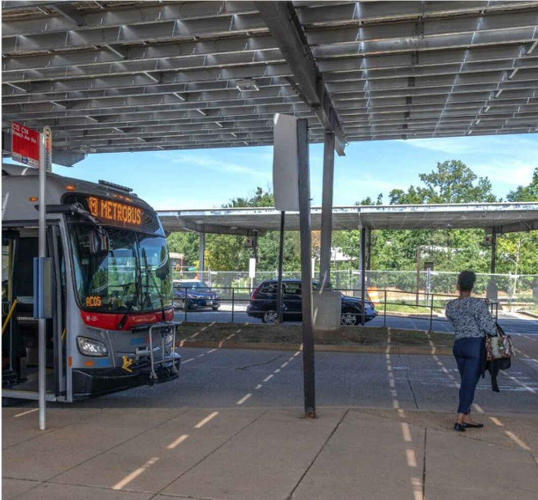
Solar Installation at Naylor Rd
