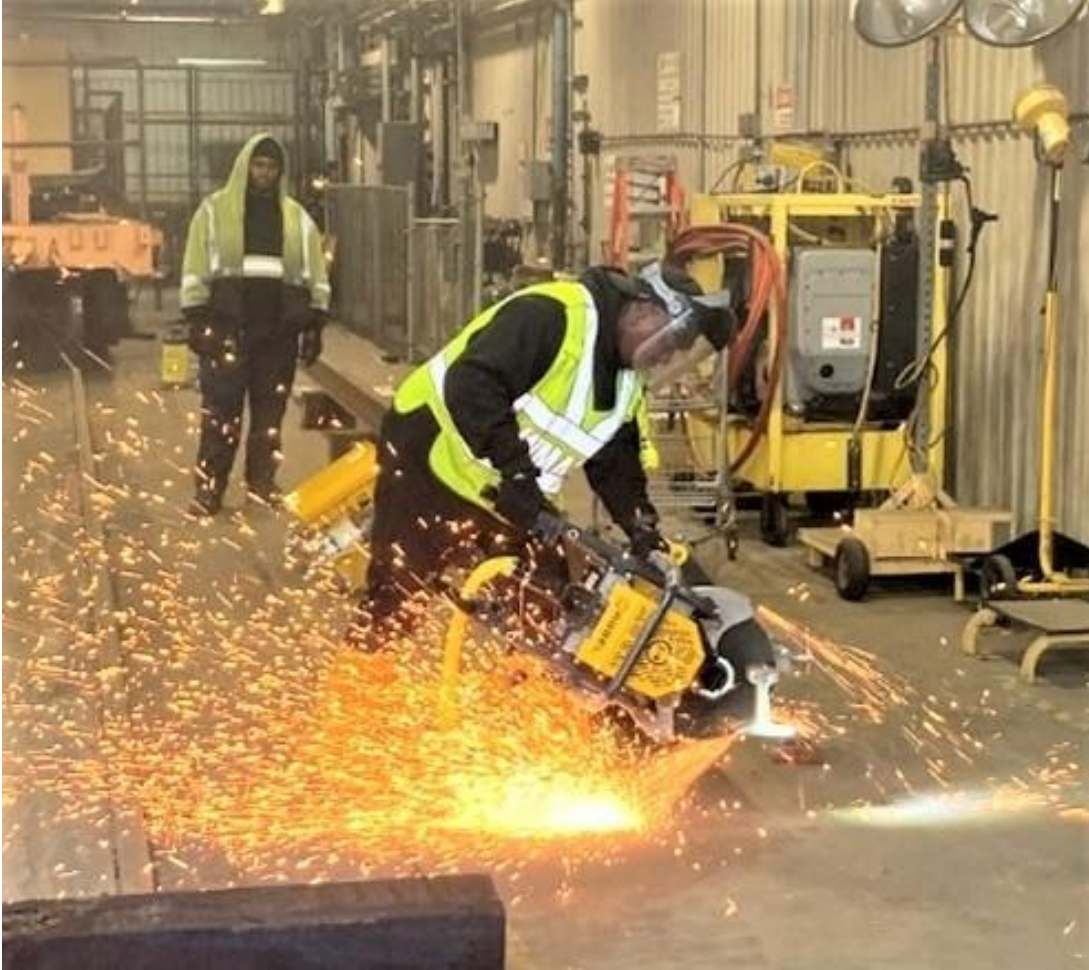
Testing battery-powered track maintenance equipment
