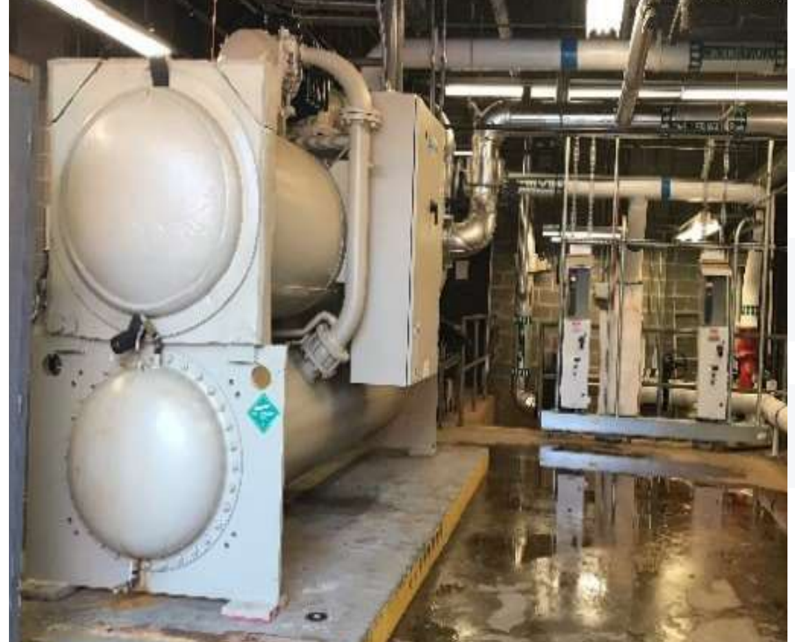
Newly Installed Chiller at Benning Rd
