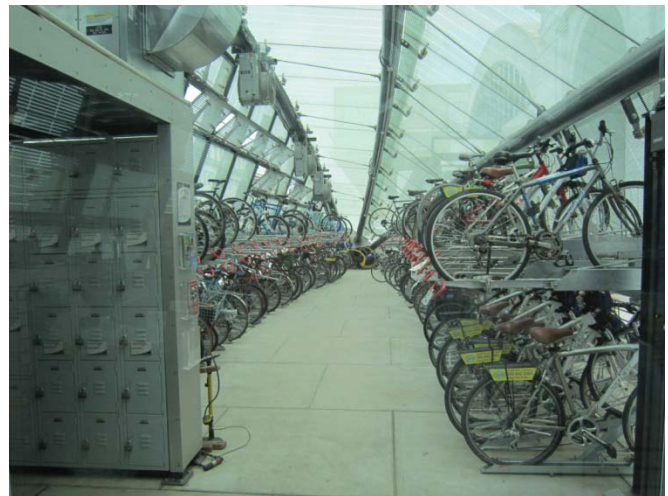
Figure 9: DC Bike Station Interior
