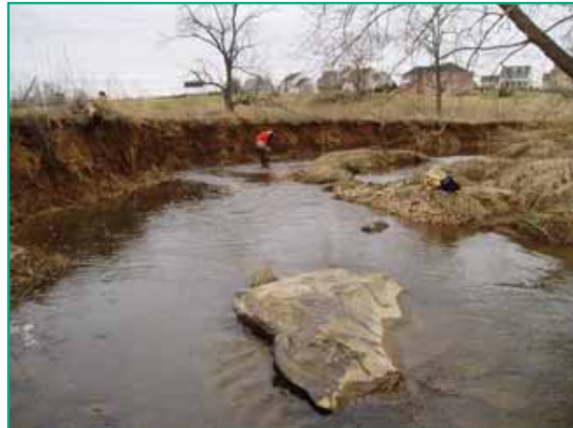
Middle Tributary - Brens Creek - (X-2) - Severe Stream Bank Erosion
