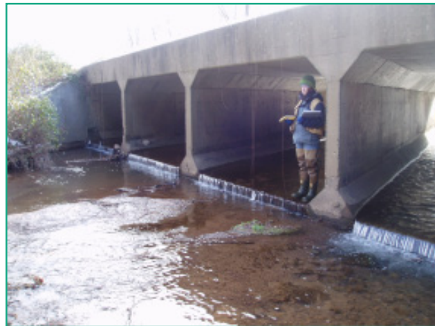
Complete Fish Barrier - Saint Clair Lane Road Culvert
