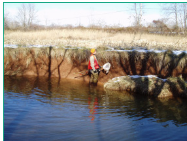
Clarks Run (Upstream of X-3) - Moderate Streambank Erosion
