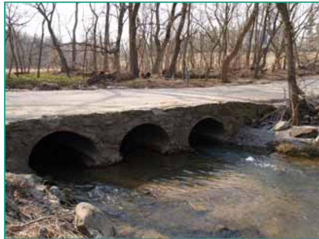
South Fork Catoctin Creek - Alder School Road Culvert
